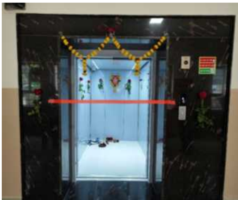
Installation of New Bed Lift Beside the Psychiatry OPD
