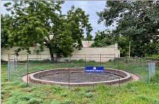
Rain Water harvesting percolation well for recharging underground water.
