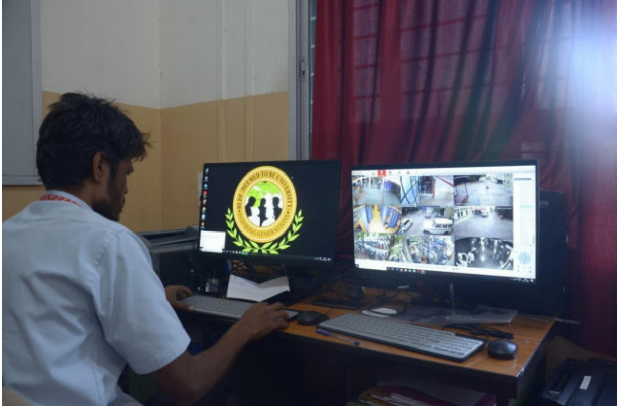
Monitoring of CCTV feed
